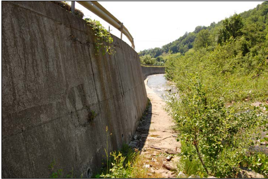
Figure 7: Frumuşeaua River concrete riverbank/completely modified.
