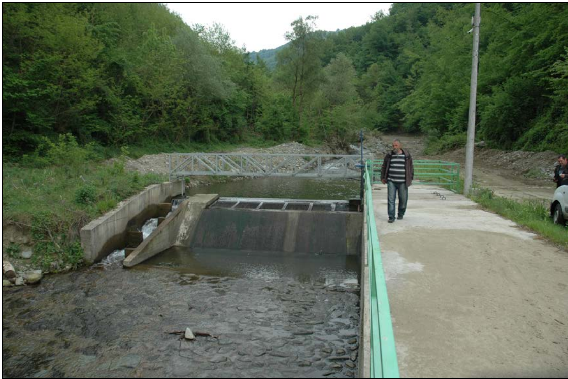
Figure 4: Garvanica water intakes of hydroelectric power plant Džep.
