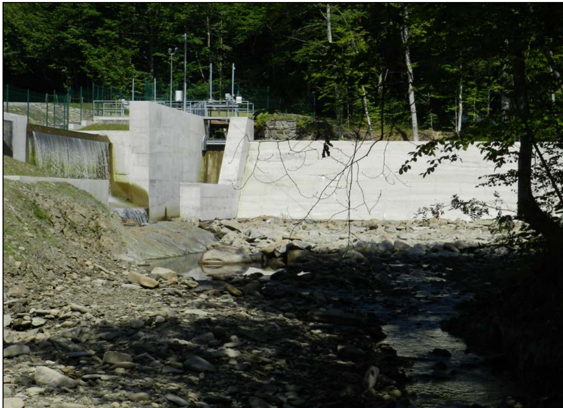
Figure 2: Tur'ya-Polianska small hydropower plant.
